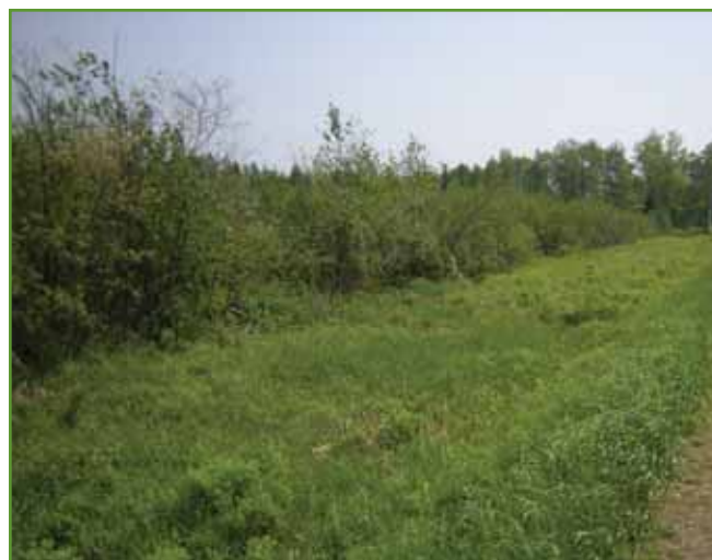
Figure 64. View of ditch near the watershed divide looking east along County Road Zz. The road grade is several feet above the surrounding terrain at this point and no maintained roadside ditch or culverts exist. Photo from USACE.
