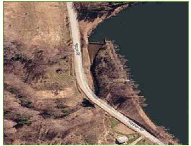
Figure 24. Silver Creek Reservoir Dam and Spillway, Parcells Corners, NY. Photo from USACE.
