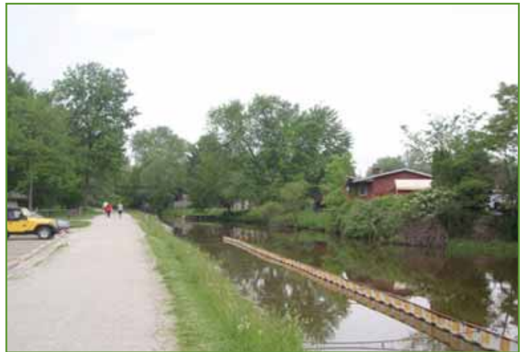
Figure 35. Typical View of Canal near Feeder Gates. Photo from USACE.
