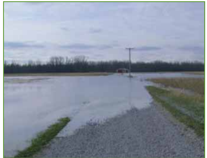
Figure 8. Flooding across the entrance road to Eagle Marsh. Photo from USACE.
