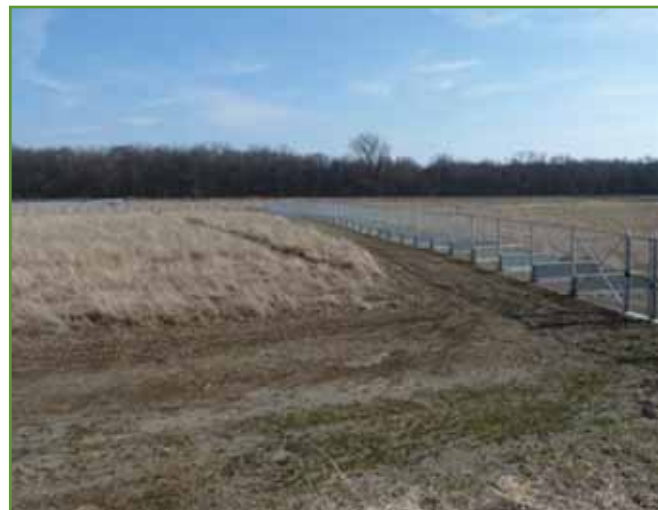
Figure 7. Photo of the temporary barrier fence. Photo from USACE.
