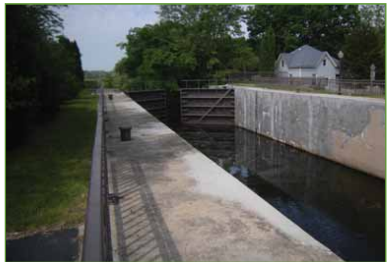
Figure 57. Portage Canal Lock. Photo from USACE.
