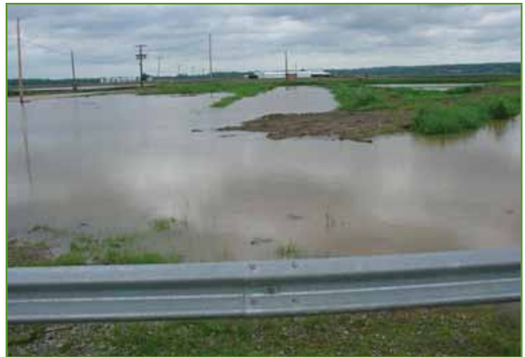
Figure 29. Flooded Area Near Willow Road and Garden Isle Road Intersection. Photo from USACE.
