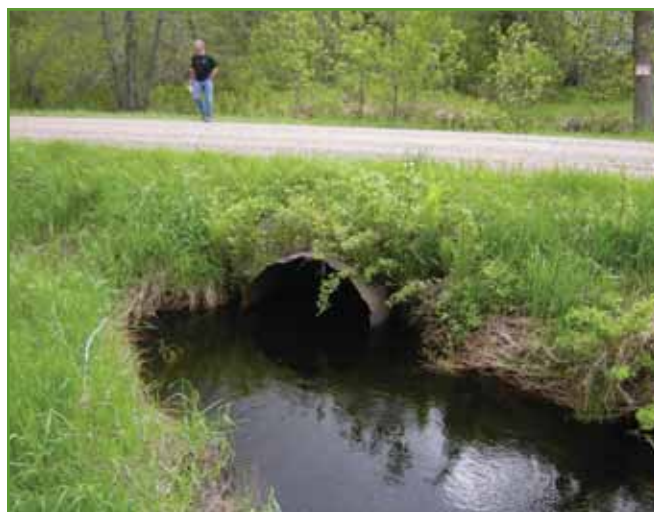
Figure 17. Southern-most culvert under 154th Avenue. Photo from USACE.
