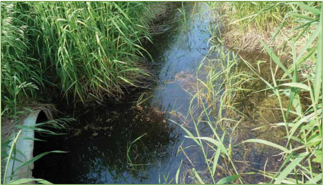
Figure 8. Photo at County Rd M, looking at the four-foot CMP on the west face (wetland side) of the Culvert. Photo from USACE in 2011.
