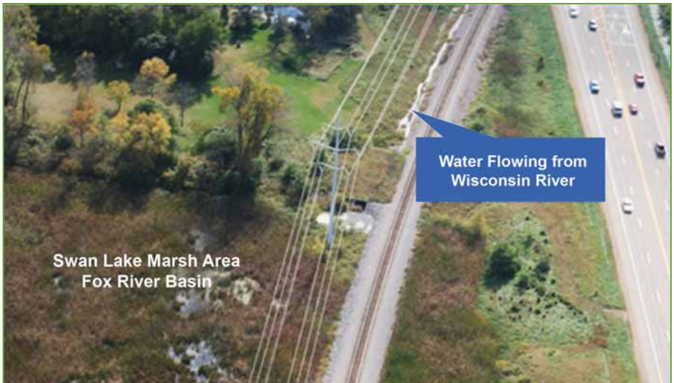
Figure 7. Aerial image of interbasin flow occurring due to backwater from Duck Creek during the September 2010 flood (10 percent annual recurrence interval flood). This image is oriented looking to the Southeast. The downstream end of the interbasin structure and pooled water in its stilling basin can be seen near the center of the photograph, just to the left of the Soo Line railroad. Imagery is courtesy of the Sand County Foundation.
