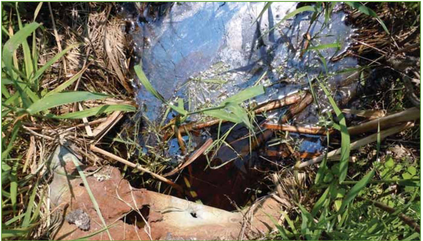
Figure 9. Willow Creek upstream face (east side) of 1.5 foot (0.46 m) CMP culvert at Lannon Rd. Photo from USACE, June 2011.
