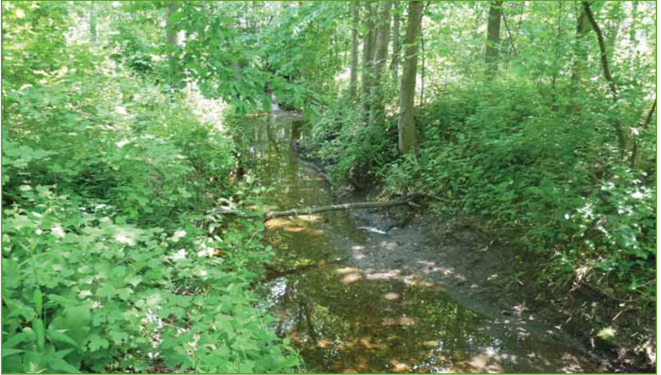
Figure 23. North end of urban storm drain near Ann Avenue (looking north). Photo from USACE, June 2011.
