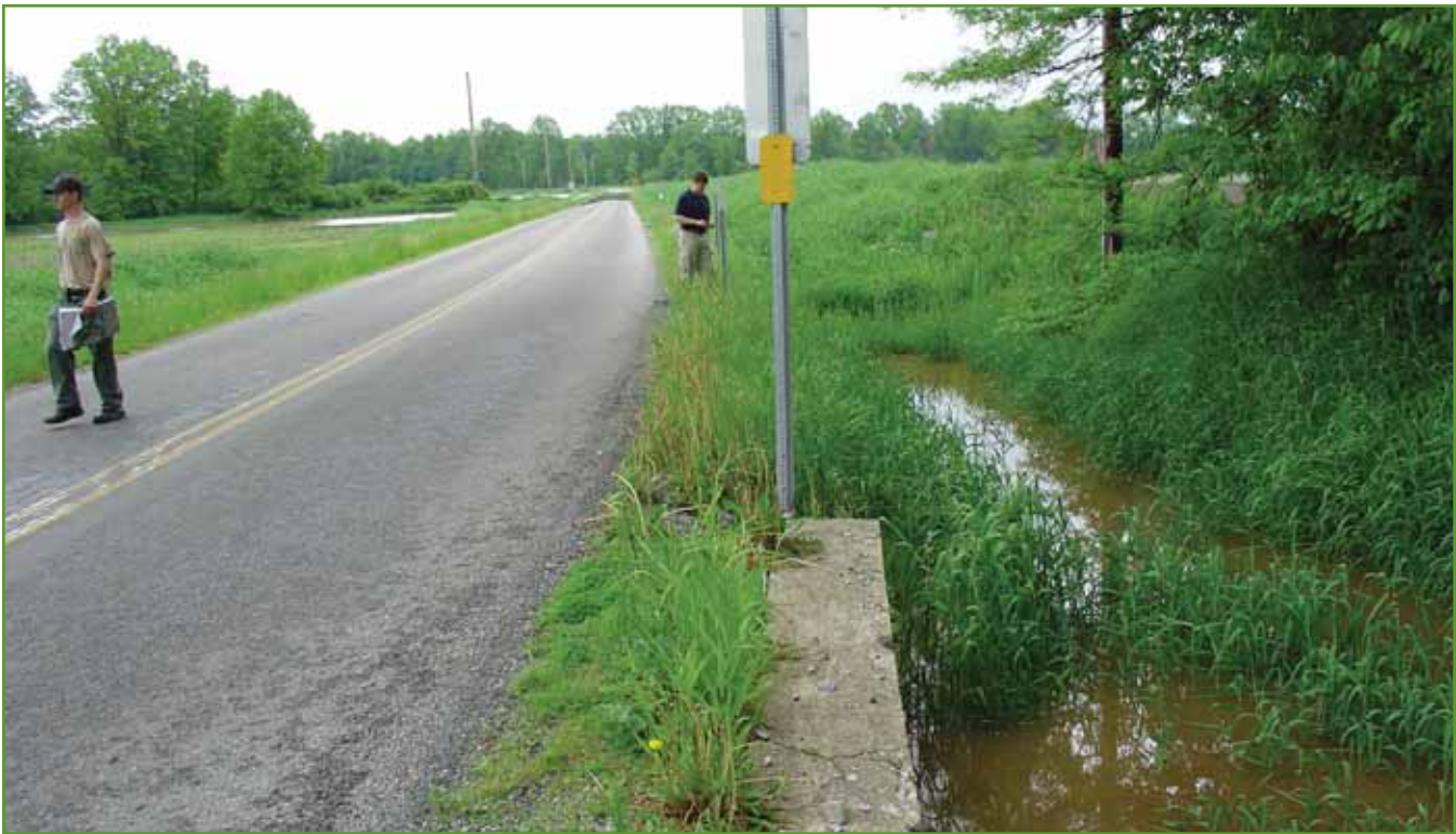
Figure 14. Roadside ditch along Franchester Road. Photo by USACE.
