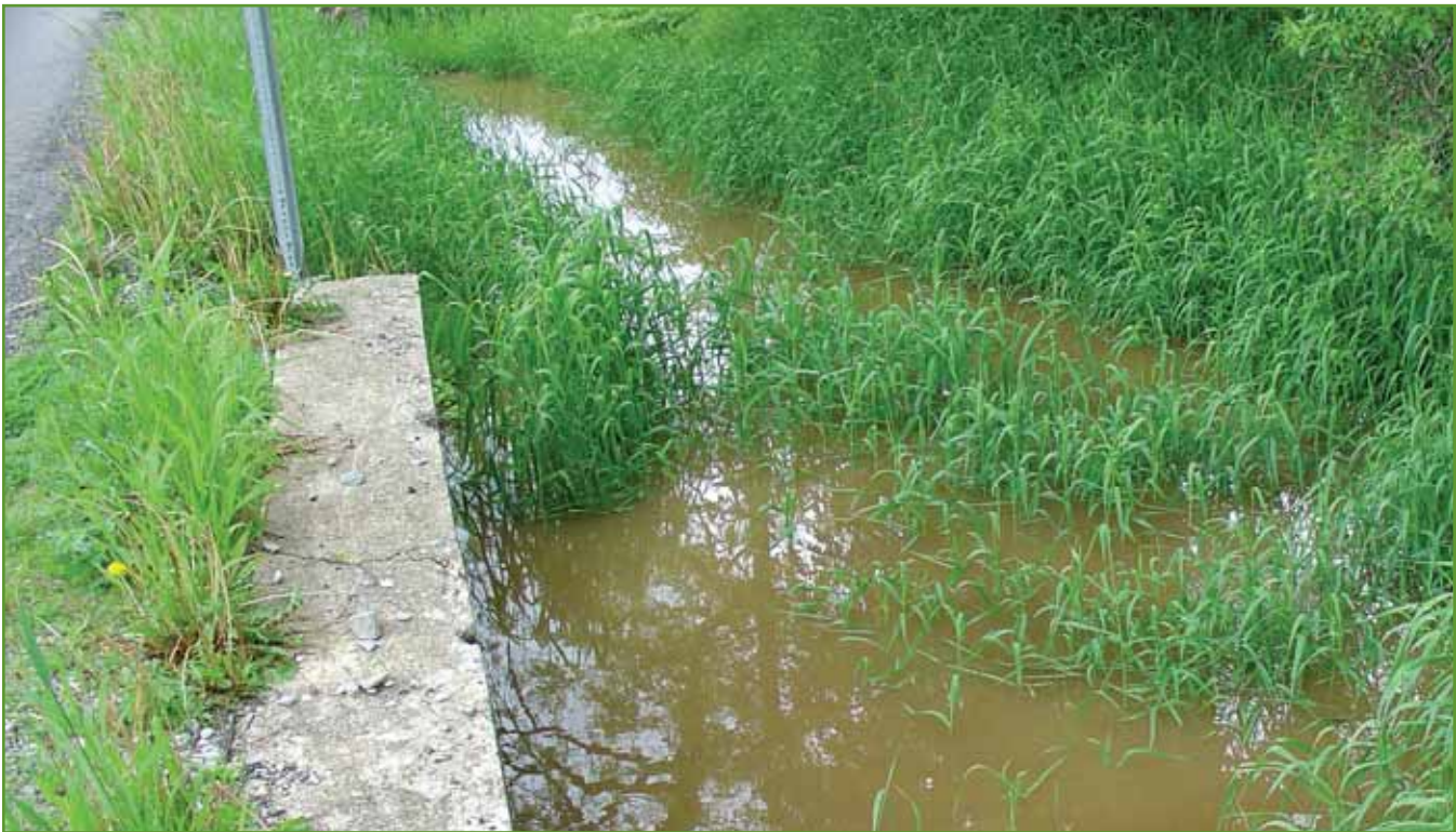
Figure 15. Storm water in ditch along Franchester Road that cross the basin divide. Close-up view of roadside ditch shown in previous figure. Photo by USACE.
