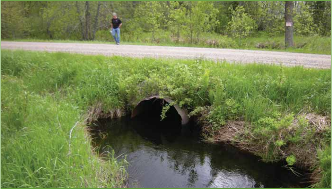
Figure 10. Southern-most culvert under 154th Ave. Photo by USACE.
