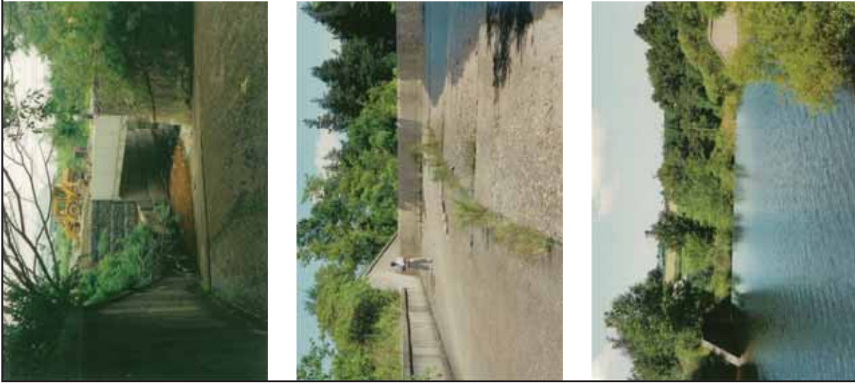
Figure 27. Silver Creek Reservoir Spillway, Parcels Corners, NY. Base of spillway shown in upper left image and spillway weir [6 feet (1.8 m) in height] shown in lower left image, with scaled profiles to the right. Pictures and profiles provided courtesy of Chautauqua County Department of Public Works. .
