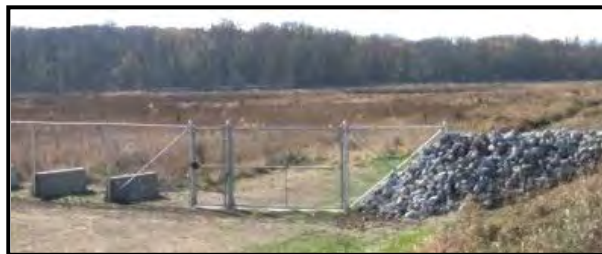
Photo 1.1: Chain-link fence ties into the Graham-McCulloch Ditch left descending berm
