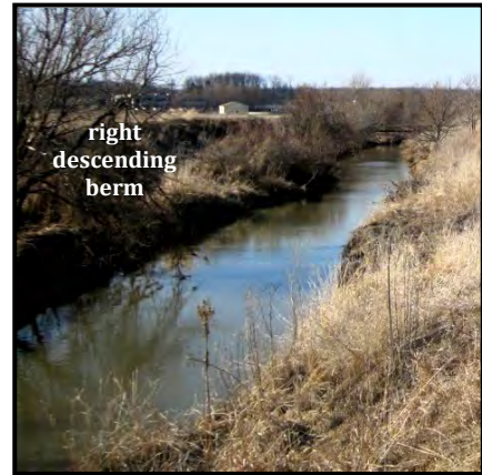
Photo 3.6: Graham-McCulloch Ditch. Proposed multi-cell wetland area will be located behind the existing right descending berm (left)
