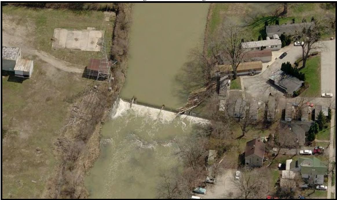
Photo 6.2: Overhead View of Huntington Dam
