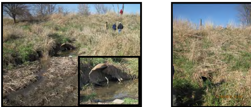
Photo 5.3 and 5.4: (Left and Right) Partially buried and abandoned culverts located in Graham-McCulloch Ditch may allow ANS movement.
