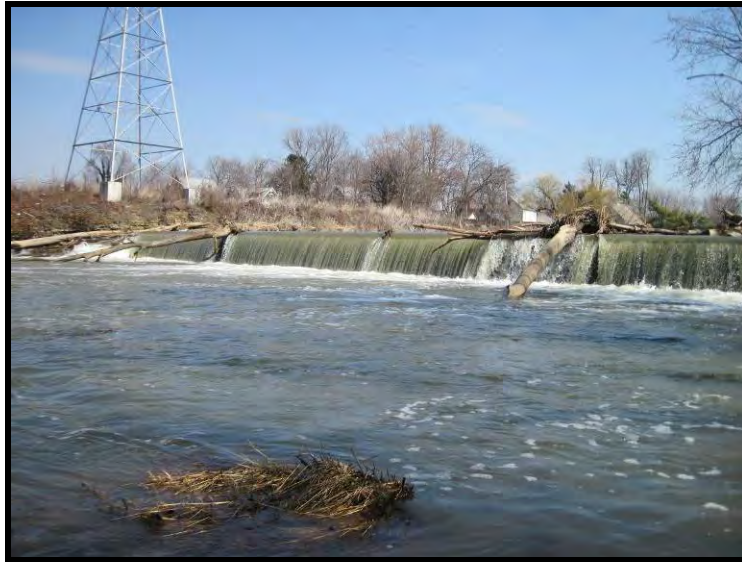
Photo 6.3: Typical Large Logs that Impact Dam
