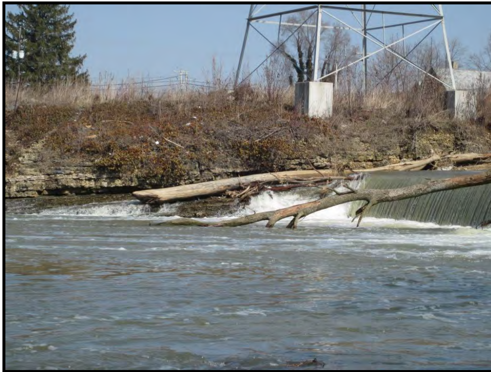
Photo 4.2: Exposed Bedrock at Huntington Dam
