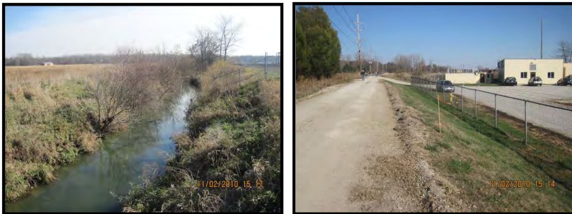
Photo 5.7: (left) Photo taken from Towpath Trail bridge looking downstream at Graham-McCulloch Ditch. The wastewater treatment plant is on right.
