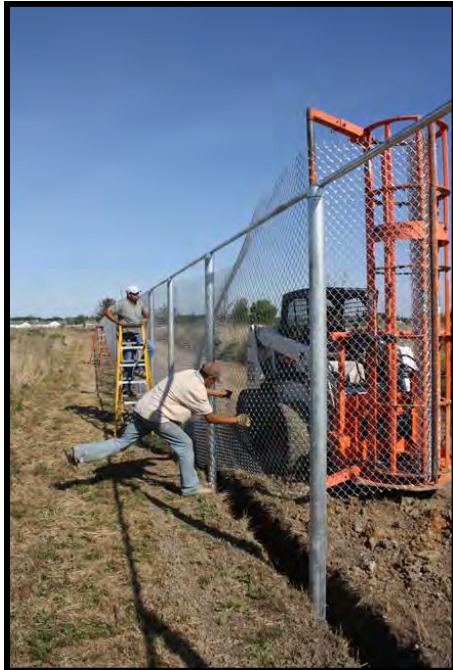
Photo 1.2: Indiana DNR fence construction
