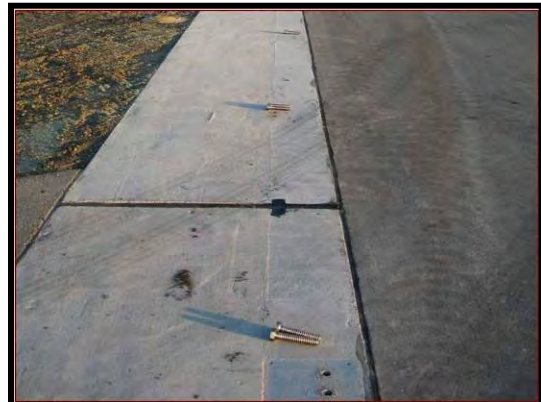
Photo 1.12: Concrete wall foundation, only bolts are visible when barrier is down
