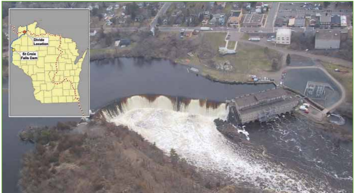
Figure 15. Hydroelectric dam on the St. Croix River at St. Croix Falls, WI. Photo from April 19, 2001. Daily river discharge was 27,500 cfs (778 cms) (USGS 05340500), a discharge between approximately a 50 percent and 20 percent chance flood event. Photo source: NOAA National Operational Hydrologic Remote Sensing Center.
