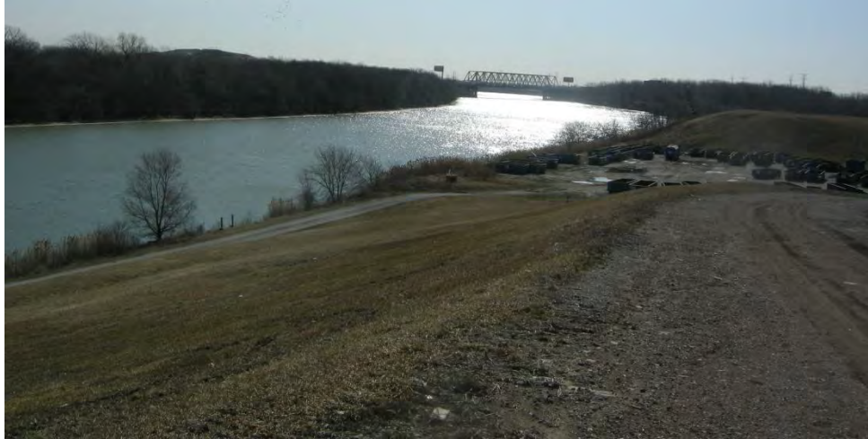
FIGURE H.2-9 View of Bishop Ford Bridge with Landfill Operations in the Foreground
