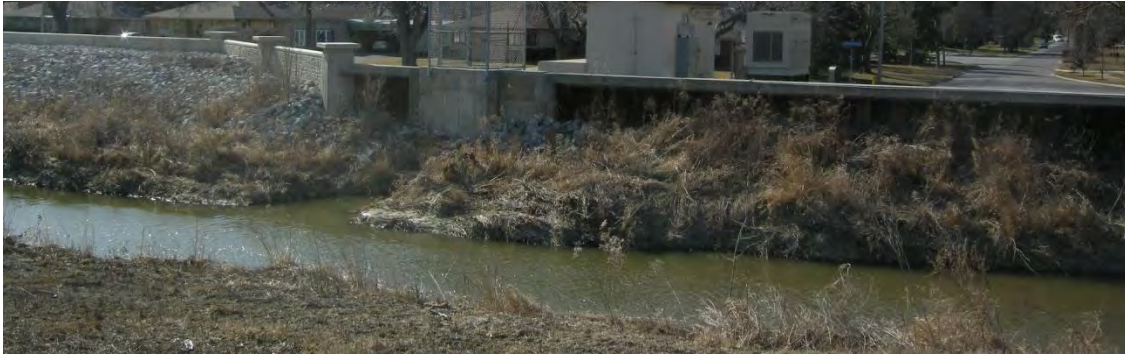
FIGURE H.2-11 Sheet Pile Observed during 30 March 2013 Site Visit
