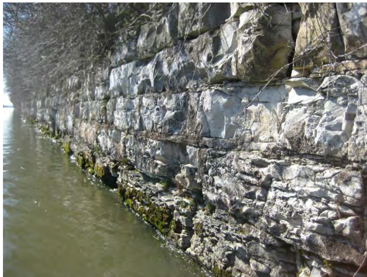
FIGURE H.2-6 Vertical Bedrock Outcrop along CSSC
