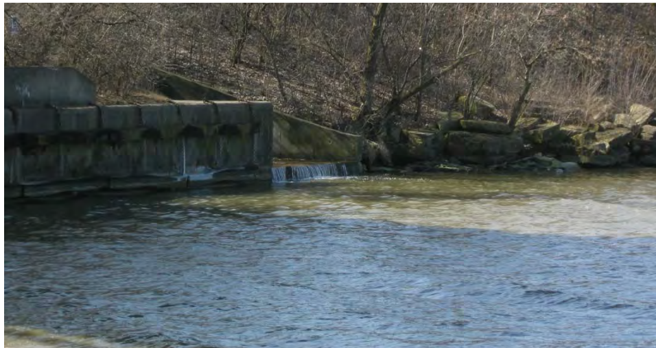
FIGURE H.2-8 Outfall in Cal-Sag Channel
