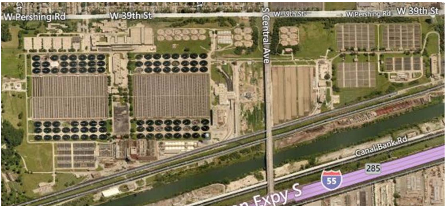
Figure 12. Stickney Waste Water Reclamation Plant
