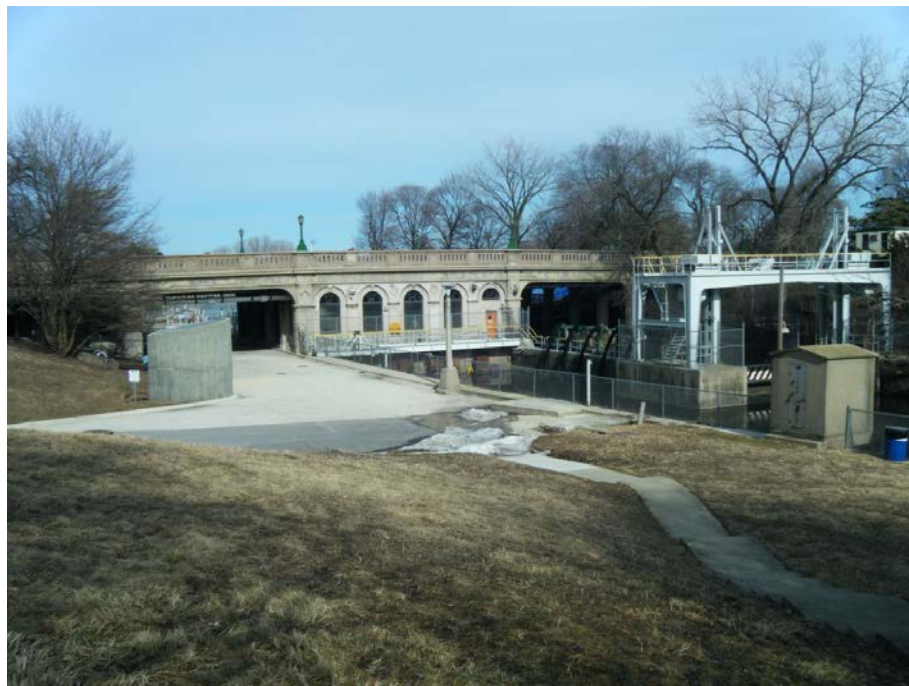
Figure 8. Wilmette Pumping Station
