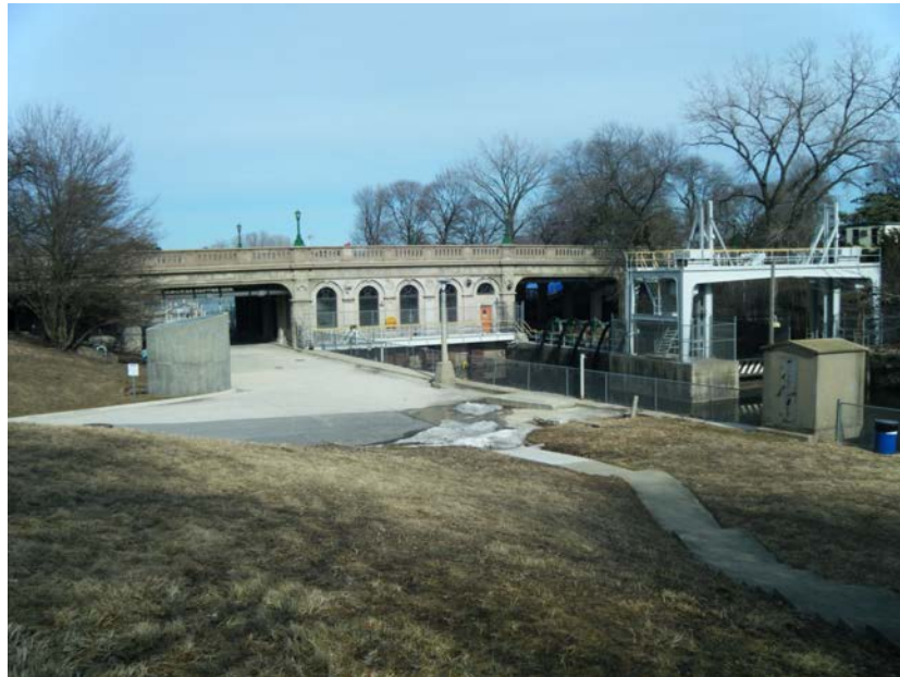
Figure 8. Wilmette Pumping Station
