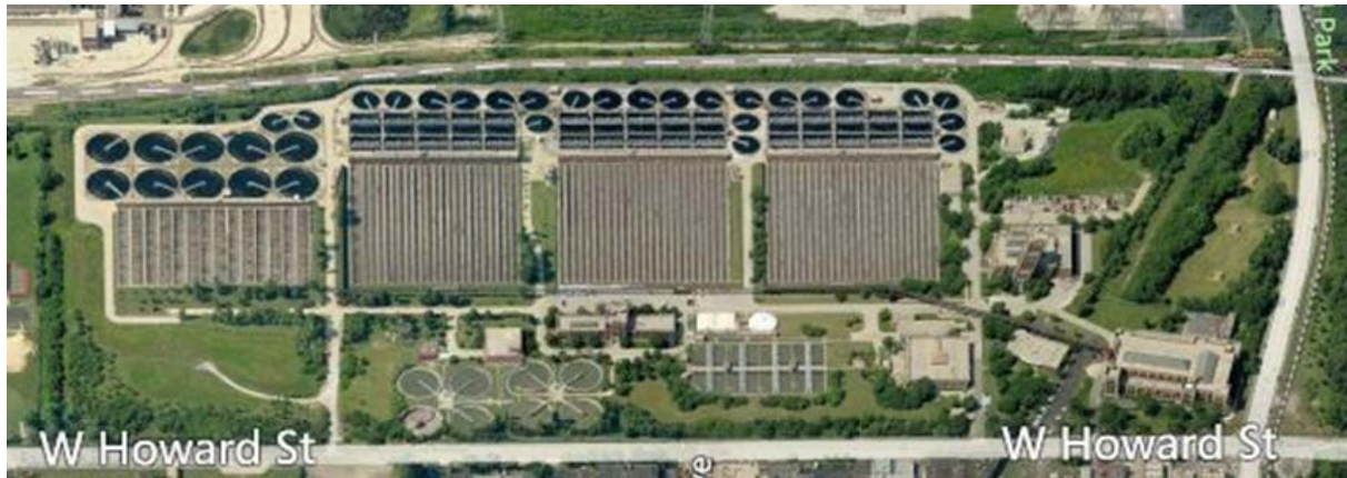
Figure 10. North Side Water Reclamation Plant
