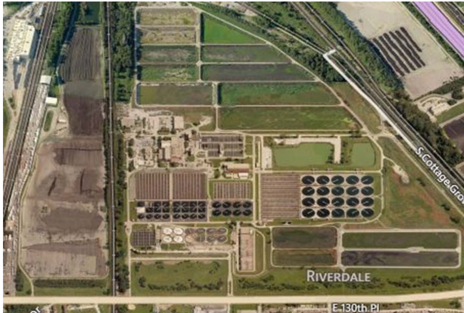
Figure 11. Calumet Waste Water Reclamation Plant
