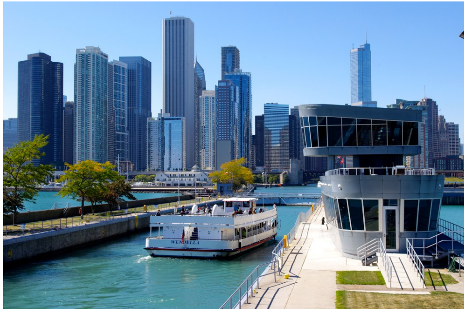
Figure 4. Chicago River Controlling Works Lock
