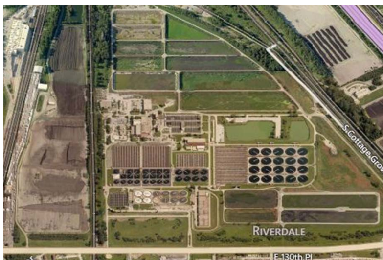
Figure 6. Calumet Waste Water Reclamation Plant
