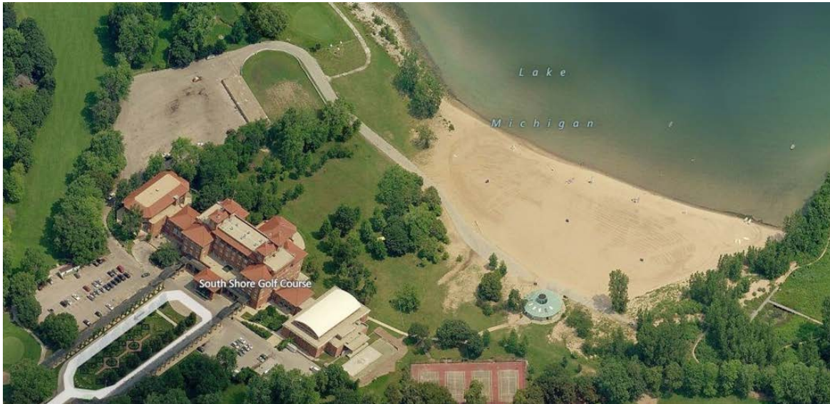
Figure 29. South Shore Beach
