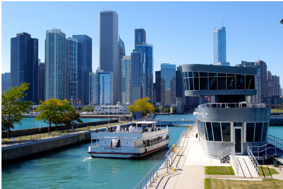
Figure 4. Chicago River Controlling Works Lock
