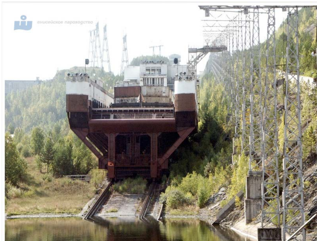
Figure 13: Barge Wet Lift at Krasnoyarsk
