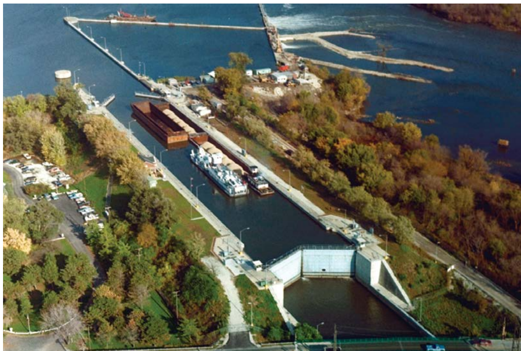
Figure 7. Brandon Road Lock & Dam
