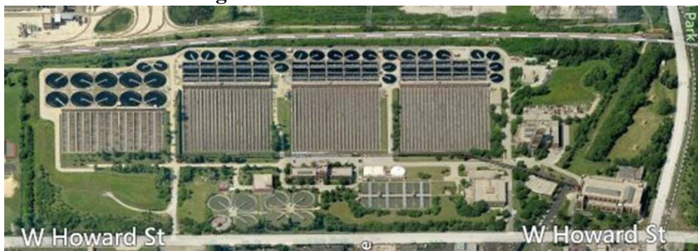
Figure 5. North Side Water Reclamation Plant
